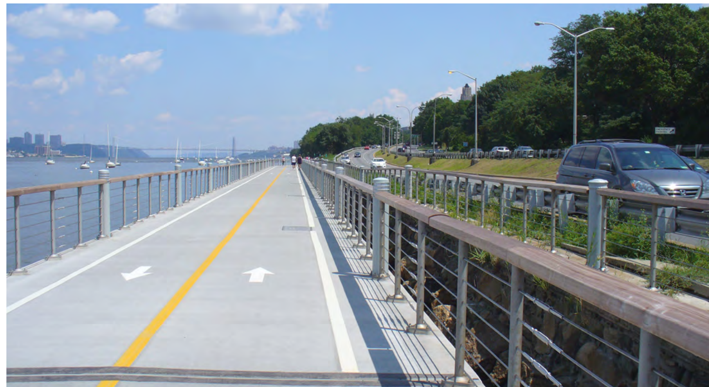
Pile supported pathway in Riverside Park, Manhattan
