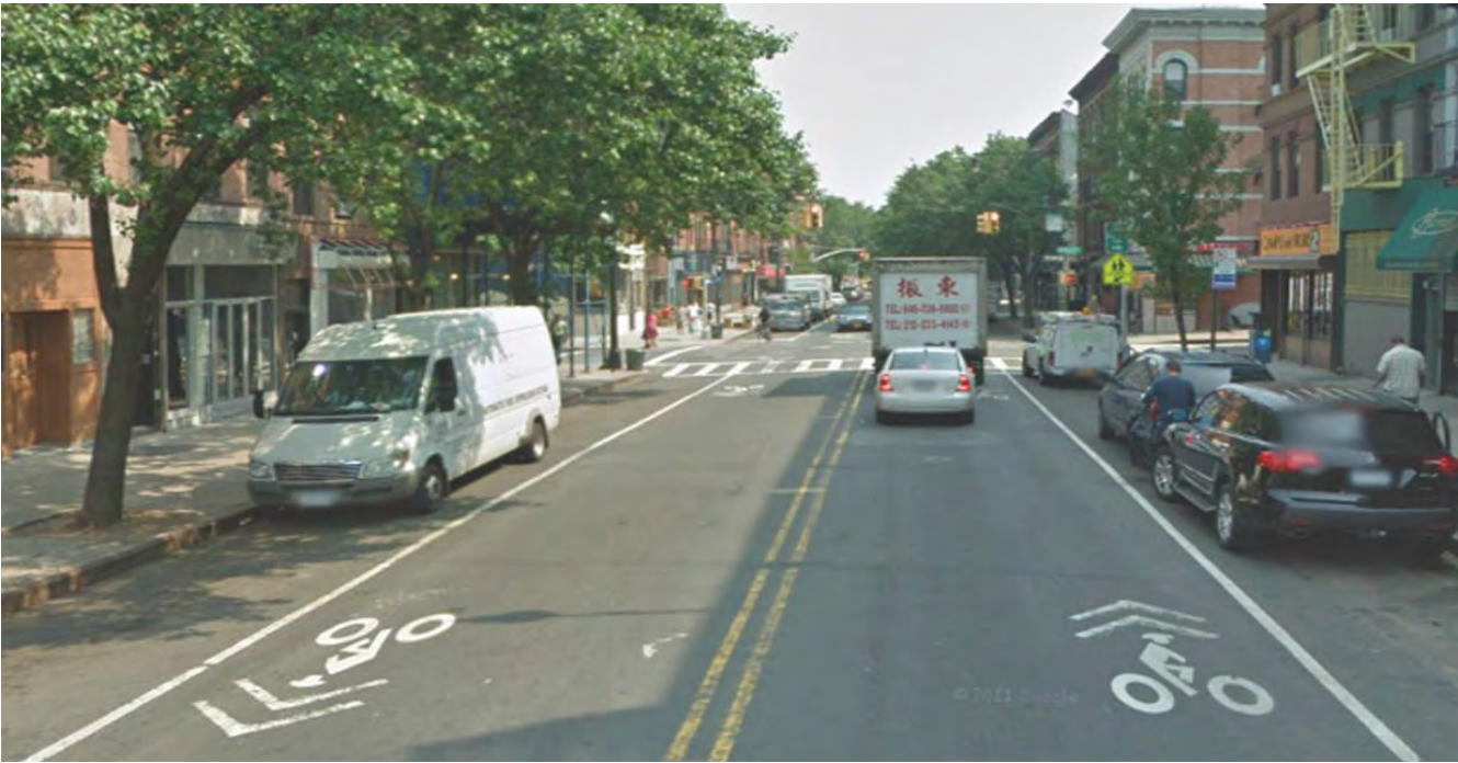
Shared Lane Markings on Fifth Avenue, Brooklyn
