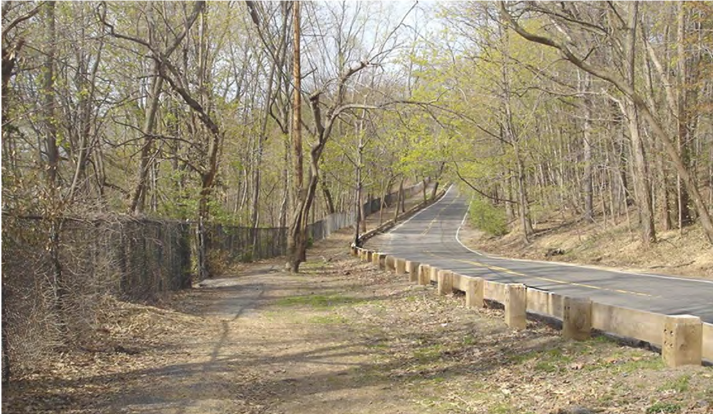
Existing Photo Palisade Avenue - BEFORE
