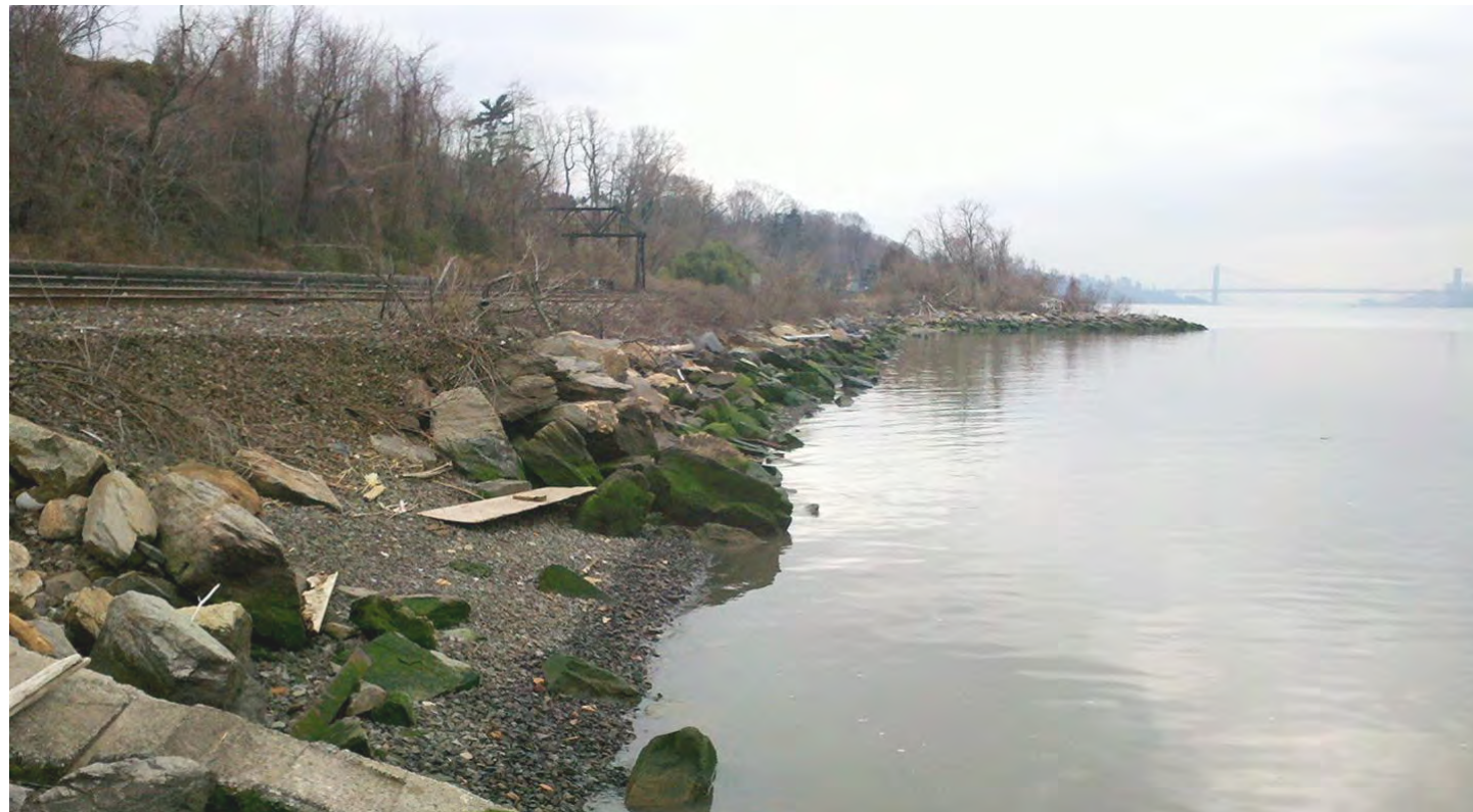
Existing Condition: Eroded Shoreline north of Riverdale MNR Train Station
